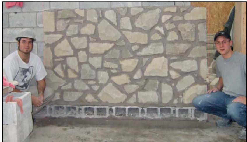
When fully cured this bagged joint blends into the stone giving a very rustic look.
