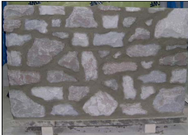
When fully cured this bagged joint blends into the stone giving a very rustic look.
